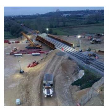
604T bridge structure; Skid Length 62m in 109 mins
