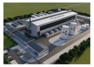
Gigastack is a large UK electrolytic hydrogen project which has been led by a consortium of Phillips 66 Limited and Ørsted (UK) Limited. The project would harness offshore wind to power electrolysis and produce hydrogen, a low-emission fuel, to power industry.
