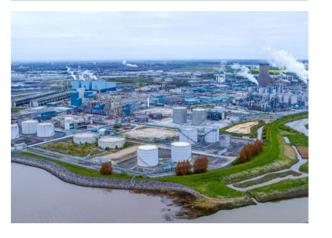
Zero Carbon Humber's kick-starter project, this flagship low carbon hydrogen production facility with carbon capture will fuel switch Triton Power station and reduce the emissions of local chemicals manufacturers.
